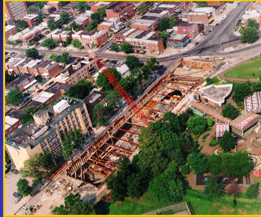
Construction of CAVF
